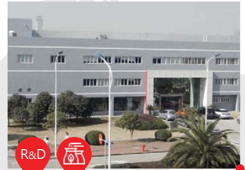
TCAC – PRODUCTION FACILITIES
