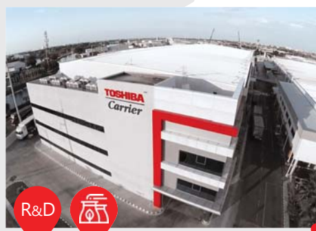
TCTC – ENGINEERING CENTRE
