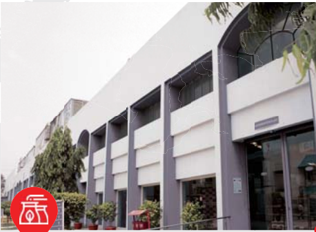
TCAI – PRODUCTION FACILITIES
