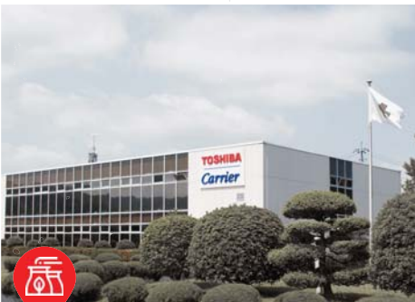
TCC – PRODUCTION FACILITIES
